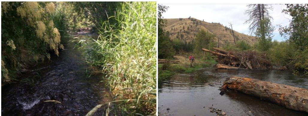
Figure 7. Restoration implemented in Project Area 14 included the creation and reconnection of side-channels (left photo) and installation of LWD structures (right photo). Photos courtesy of the SRSRB.
