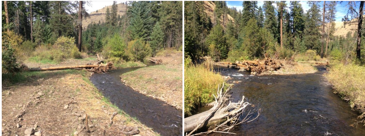
Figure 3. Restoration implemented in Project Area 1 included the creation of side channels and addition of LWD structures. No CHaMP site is present in this Project Area. Photos courtesy of the SRSRB.
