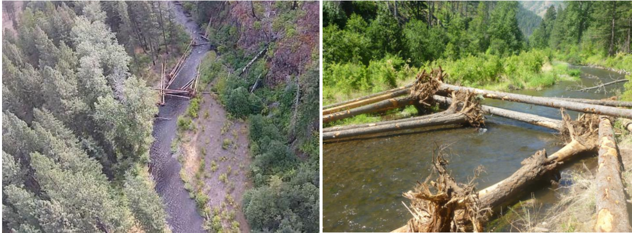
Figure 4. Restoration in Project Area 3 included the addition of LWD by helicopter. Photos show LWD structure located in CHaMP site 519039. Aerial photo courtesy of the Pomeroy Conservation District.
