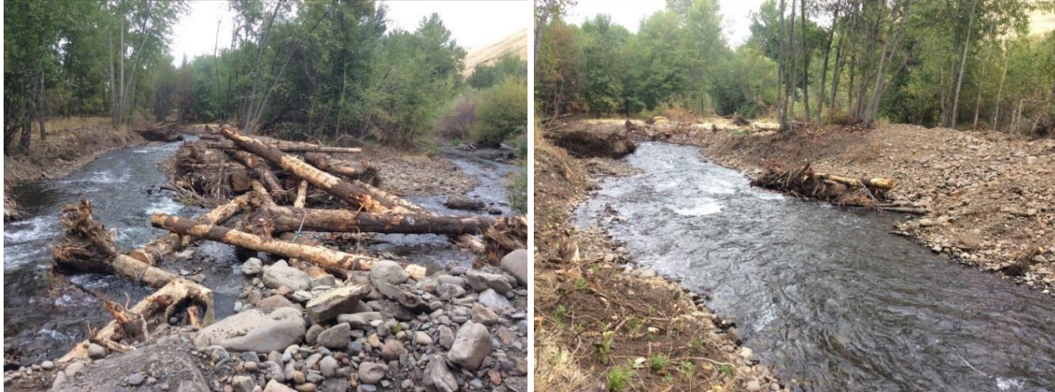
Figure 8. Restoration implemented in Project Area 15 included the installation of LWD structures (left photo) and the creation of new side channels (right photo). Photos courtesy of the SRSRB.
