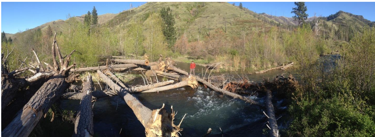
Figure 5. Restoration implemented in Project Area 10 included the addition of LWD.
