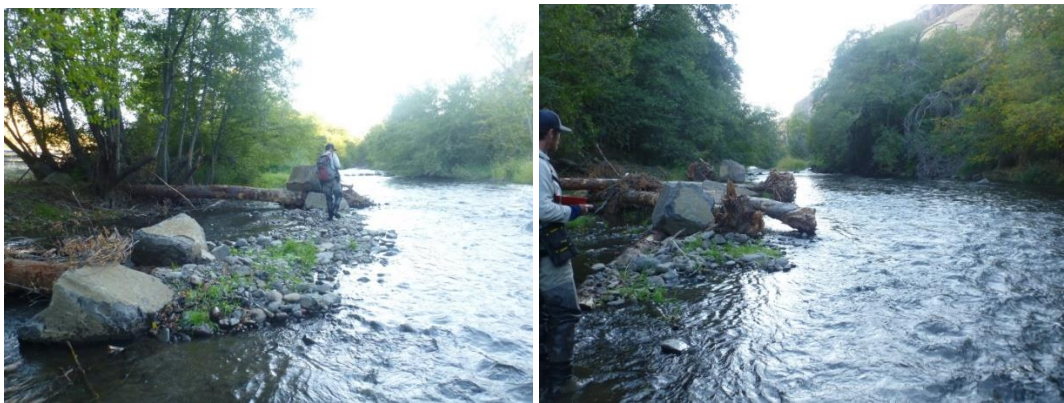
Figure 9. Photos showing two of eight LWD structures placed in Project Area 22. CHaMP post-treatment sample not available for this report.
